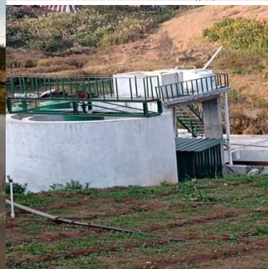
BORE WELL WATER
